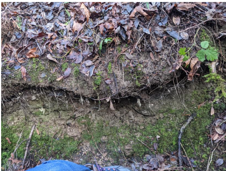
Figure 6 – Undercutting of ditch bank
