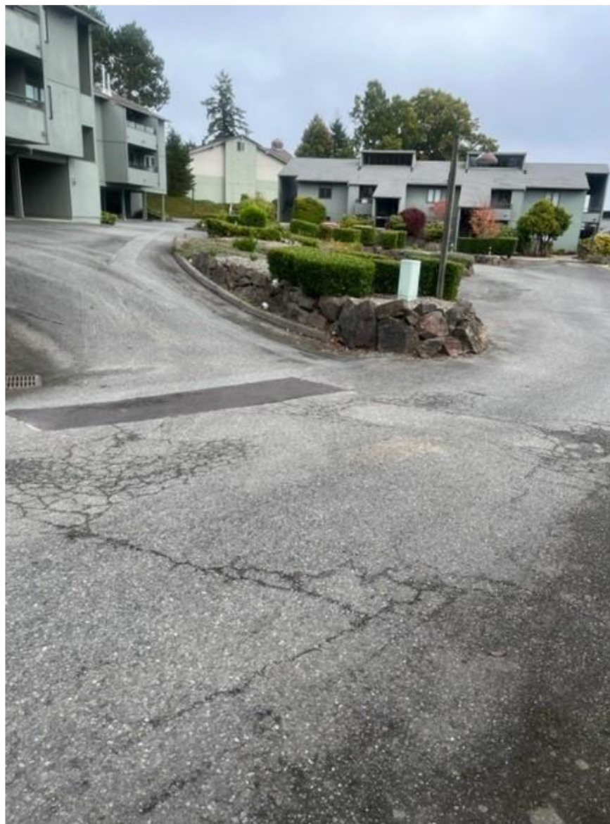
Catch Basins at Entrance to Building 13
