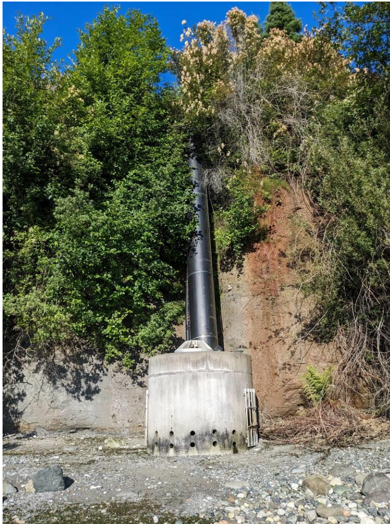
Libby Court Outfall – July 13, 2023
