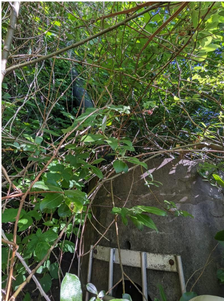
Pope Way Outfall Structure Inlet Pipe – July 13, 2023
