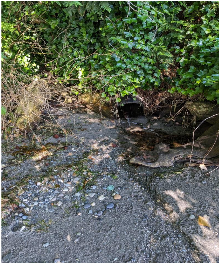
Montgomery Court Outfall (Between 192 and 200 Montgomery Court) – July 13, 2023
