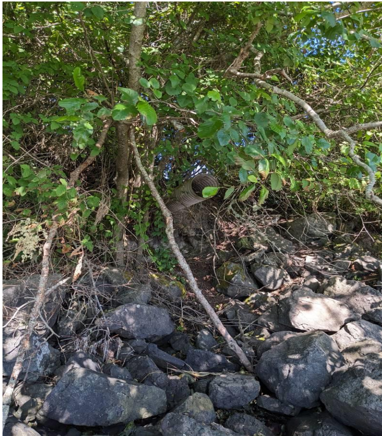
Wastewater Treatment Plant Drainage Outfall – July 13, 2023
