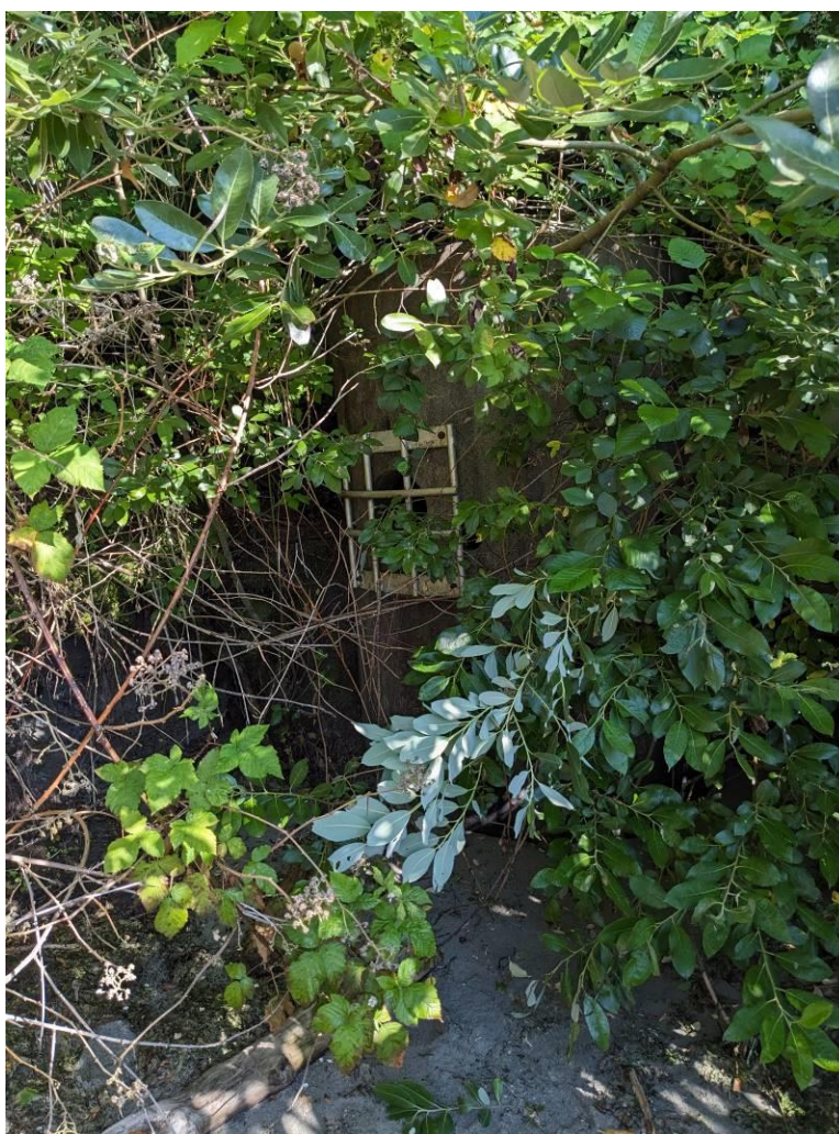
Pope Way Outfall Structure – July 13, 2023
