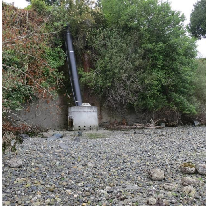
Libby Court Outfall – July 13, 2017
