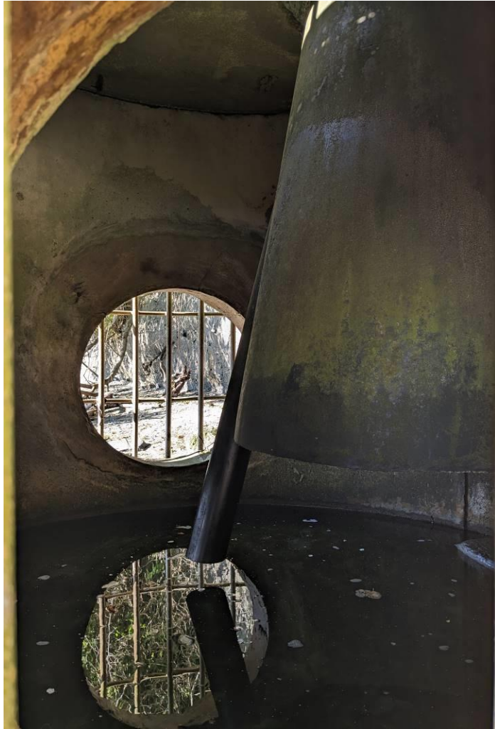
Libby Court Outfall Interior – July 13, 2023
